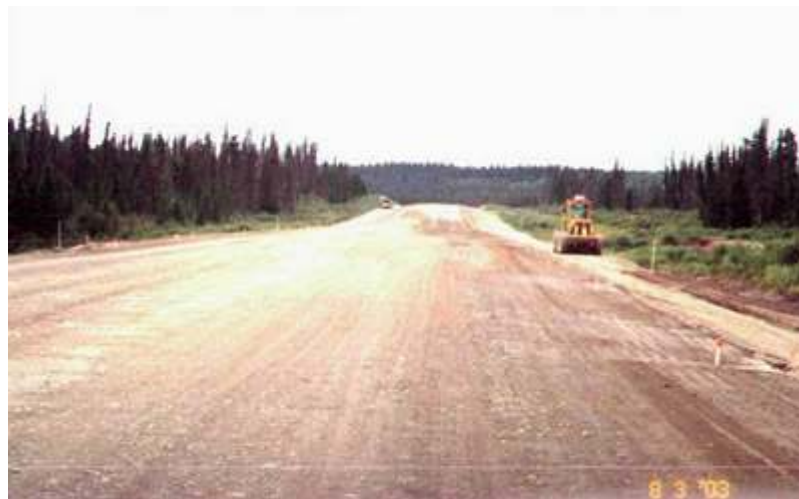
Typical Construction Zone on the Alaskan Highway
